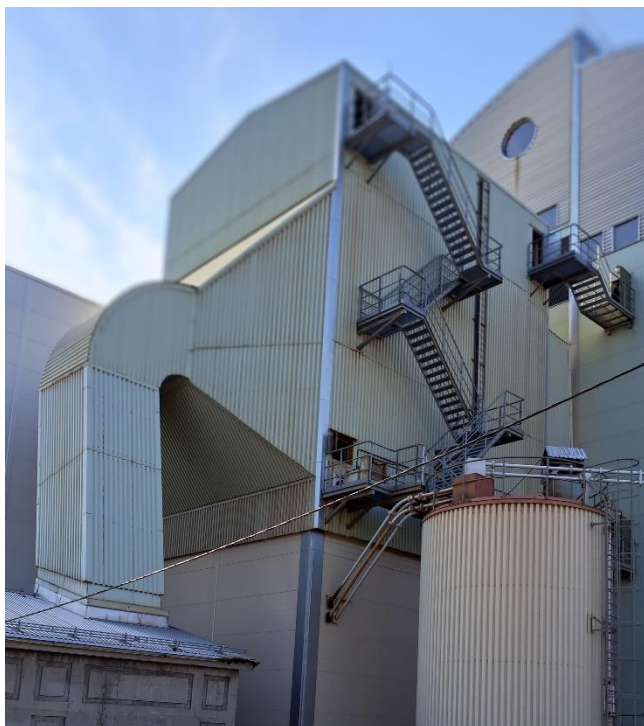
Existing ESP to be replaced with ANDRITZ ESP
